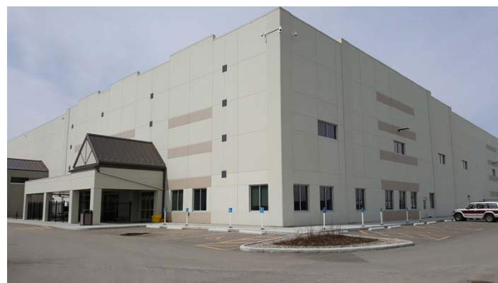
Home Depot Distribution Centre, Calgary, AB
