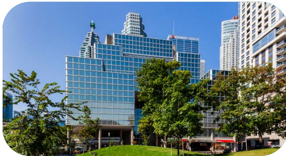
33 YONGE STREET, TORONTO, ON The Outstanding Building of the Year (TOBY) Award (500,000–1M ft 2 ) – BOMA Canada
