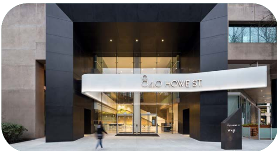
840 HOWE STREET, VANCOUVER, BC The Outstanding Building of the Year (TOBY) Award (Renovated Building) – BOMA BC
